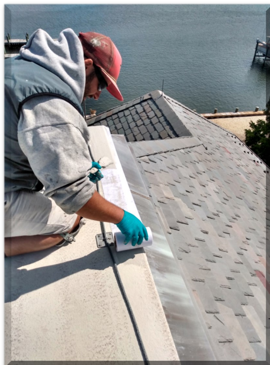
Addressing all the critical areas with Fabric Reinforcement to assure a leak free roof.
