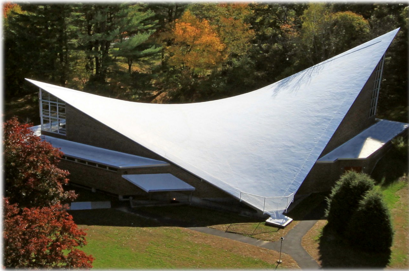
The completed Acrylabs System enhances the roof's unique curves and features
