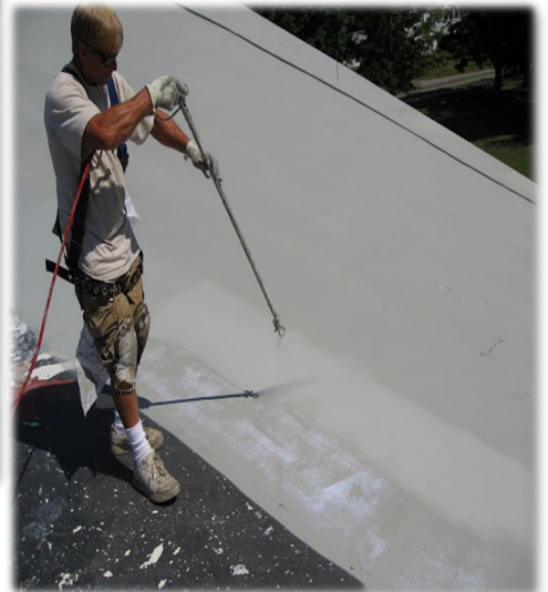
Experienced applicator using a spray technique to embed Fabric Reinforcement
