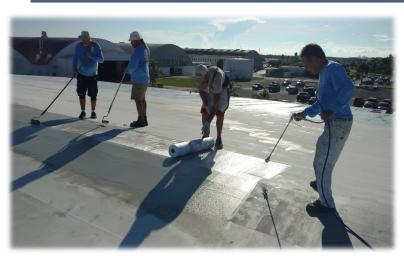
**Spray Technique Installing Fabric**
