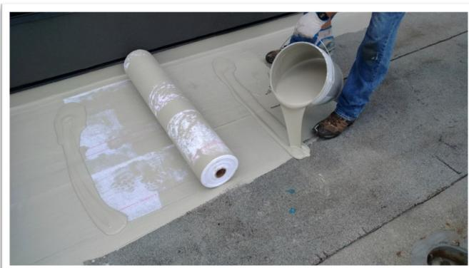
The A.L.A.R.M. - System can be applied to concrete, plywood, OSB, EPS, fiberglass, cement board, asphalt, BUR, modified bitumen, EPDM, single-ply membrane systems, and metal.
