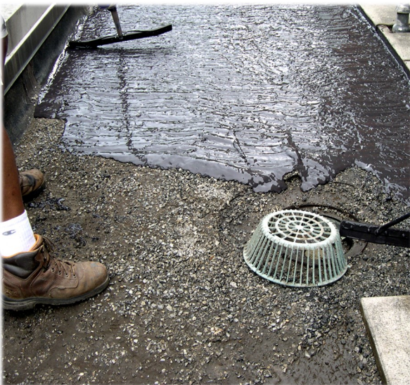
Applying Asphalt Emulsion
