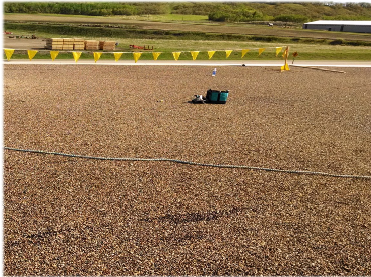
Worn out Tar and Gravel with Asphalt Emulsion ready to be installed
