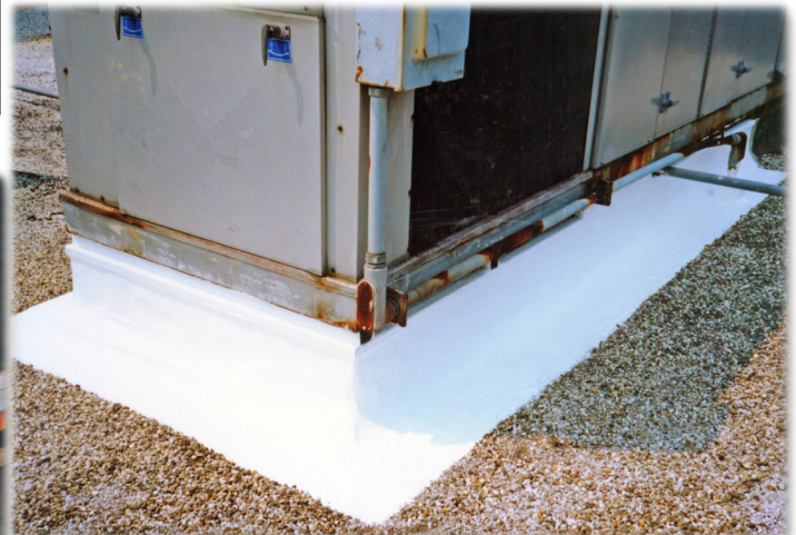
The Acrylabs Patch Kit was the perfect tool for making the repair and creating a watertight curb
