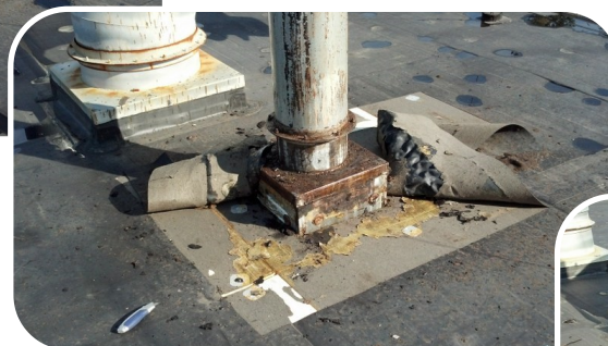
Removing damaged EPDM to expose ISO board
