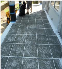
Acrycrete splatter technique knocked down with bull float
